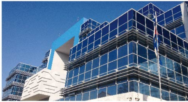
CECMED National Drug Laboratory Water-cooled Screw Chiller Hydronic Air Handling Unit Fan Coil Unit Cuba
